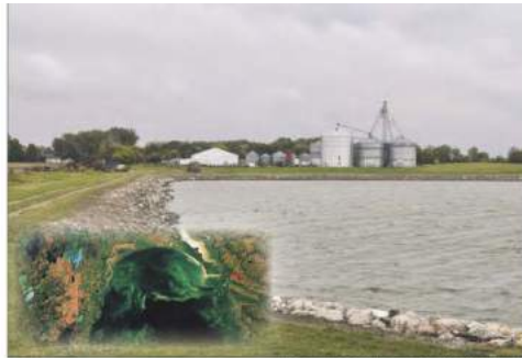
ALISA ANDERSON - DAILY NEWS - COURTESY TORACERA COMMINS Breckenridge, Minn., has a primary 80-acre wastewater retention pond, and two secondary ponds, like the one pictured. Wastewater goes into the primary pond first, then goes into the secondary pond to sit for 180 days. Inset at bottom left, an aerial view of the algal blooms in Lake Winnipeg, Canada.
